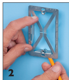
2 Bracket is template for the opening. Face out, trace the bracket along inside of bracket flange.
