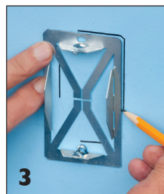
3 Turn bracket over. Use edge to complete tracing cutting guide.
