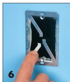
6 Bend all four corner supports into hole and around drywall to set LV15 securely in opening.
