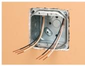
1 Place Device Support Plate on the wall opening to determine the amount of coverage needed. Select the necessary wall plate Jumbo, Mid-size or Standard.
